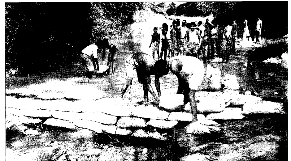
Volunteers of Satpuda Foundation work to construct a check-dam. DH PHOTO
