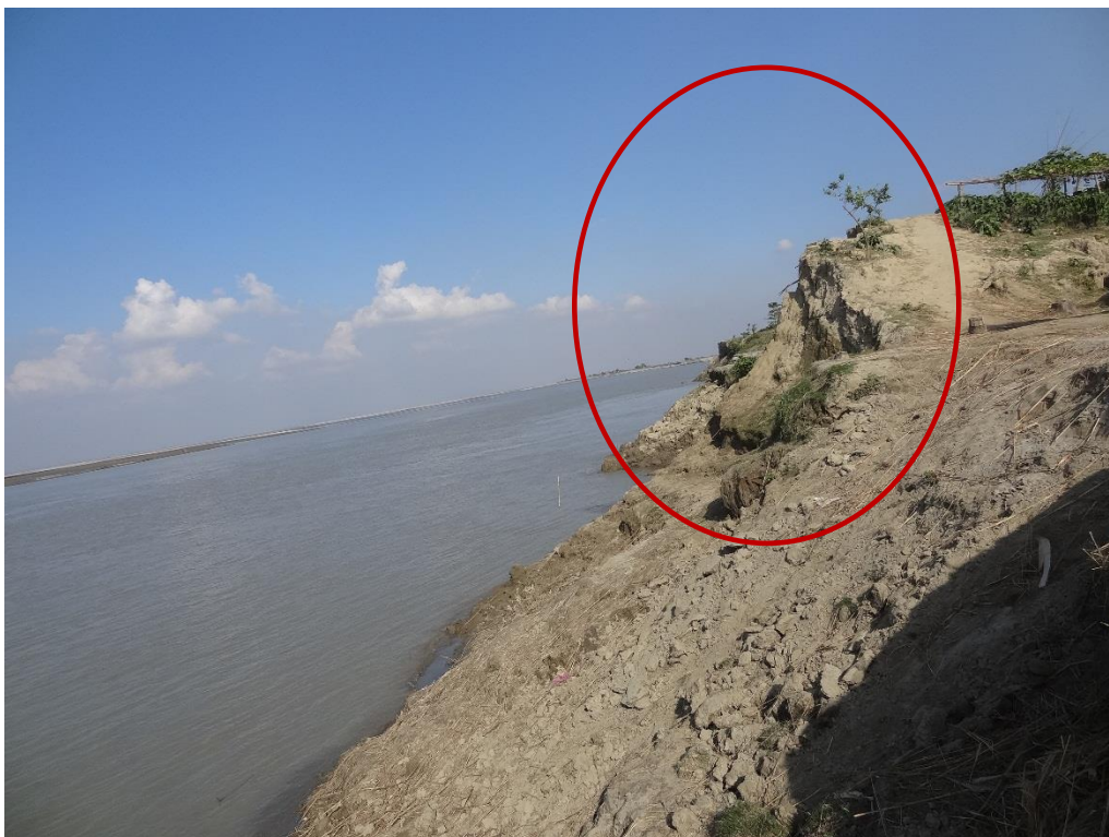
Figure 95: Eroded part of the Land spur at Lahorighat, Morigaon
