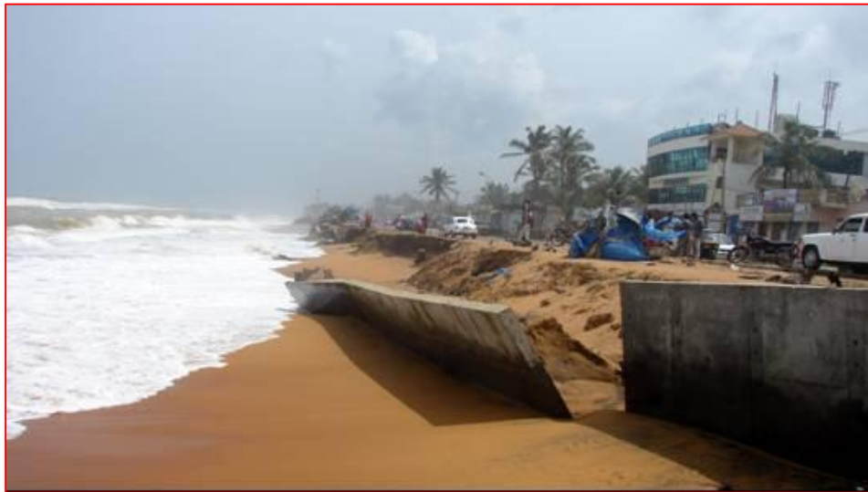
Photo 2 : Failure of Vertical Wall
