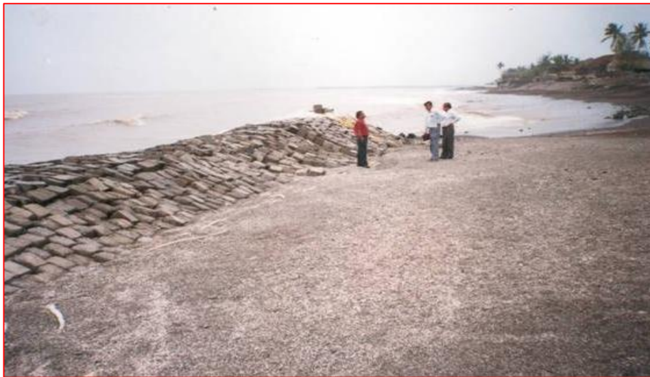
Photo 10: Discontinuity of a Seawall
