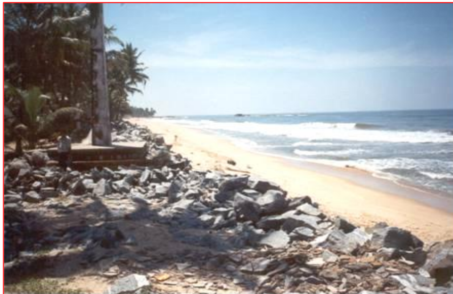
Photo 12: Rubble stones Dumped as Temporary Measure
