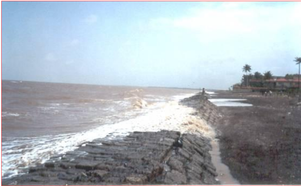
Photo 7: Overtopping of Waves Over Seawall
