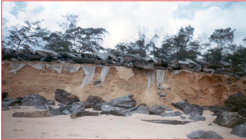
Photo 6: Inadequate Filter Layer Exposed After Damage to Seawall
