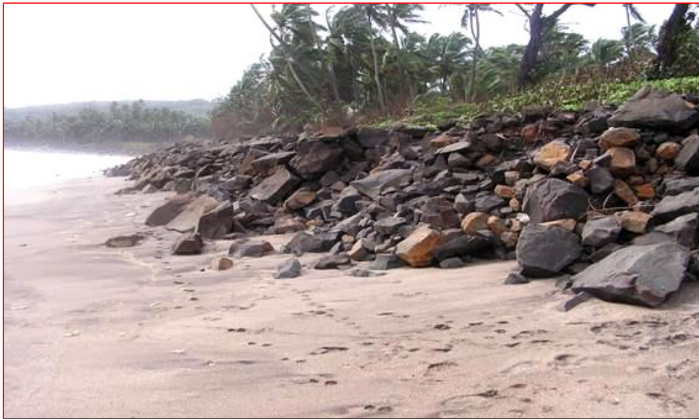
Photo 4 : Under Design of Armour layer Leads to Failure of Seawall
