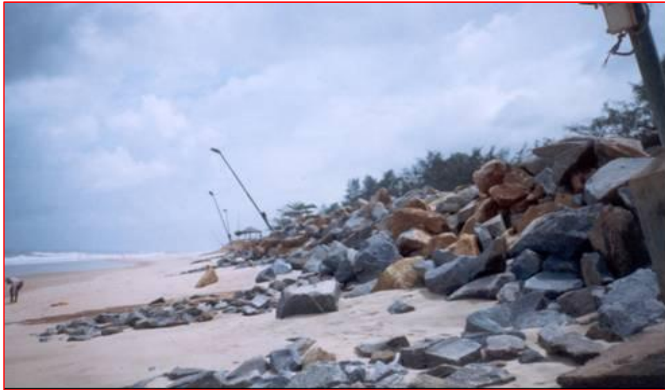
Photo 13: Damage to Seawall due to Non-maintenance
