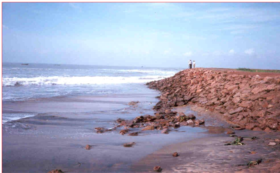
Photo 11: Revetment with Single Layer Armour
