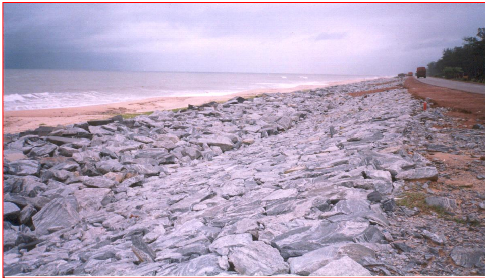
Photo 5 : Seawall With Toe Protection
