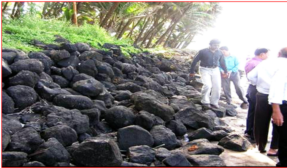
Photo 8 : Rounded Stones in Armour Layer of a Seawall
