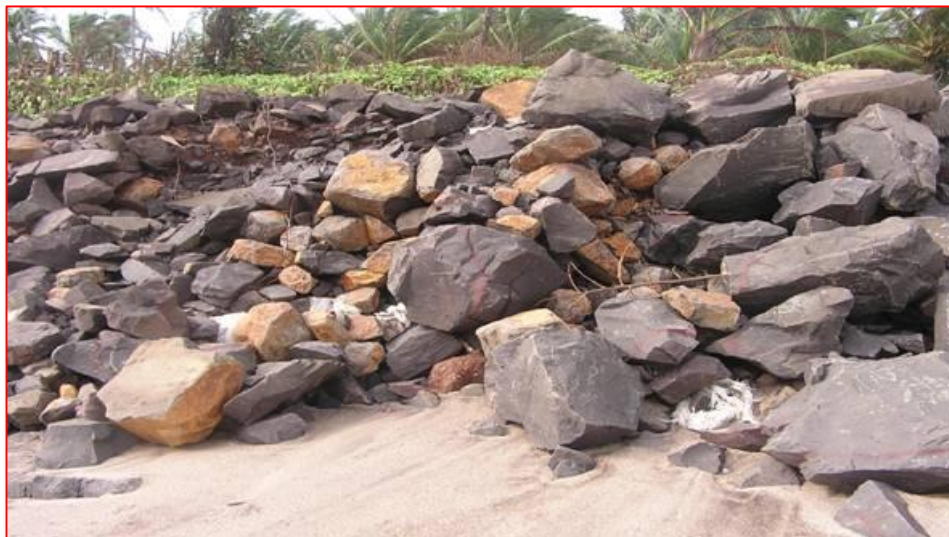
Photo 9: Pockets in Armour Layer of a Seawall
