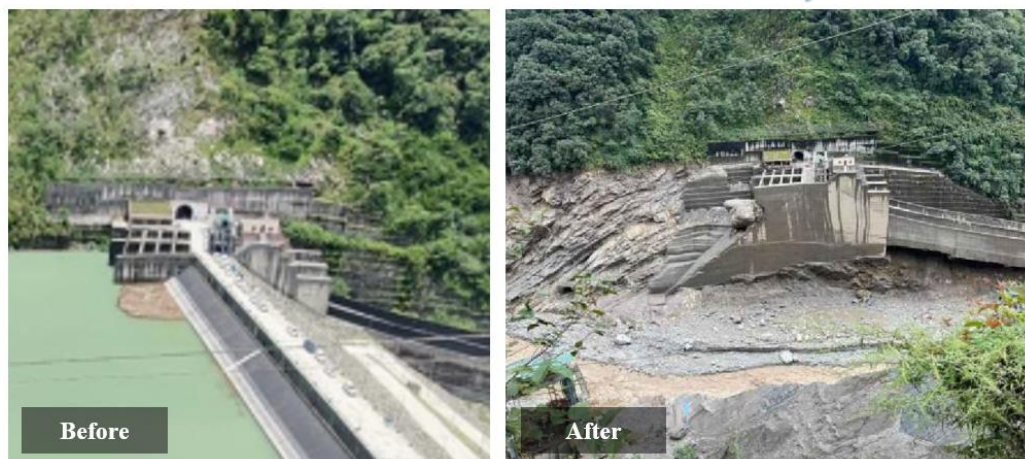
Figure 7 Depicts the Teesta-III Dam before and after the GLOF event on 04.10.2023
