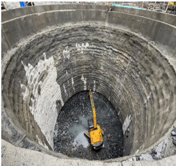
Excavation of Left Bank Vertical Shaft
