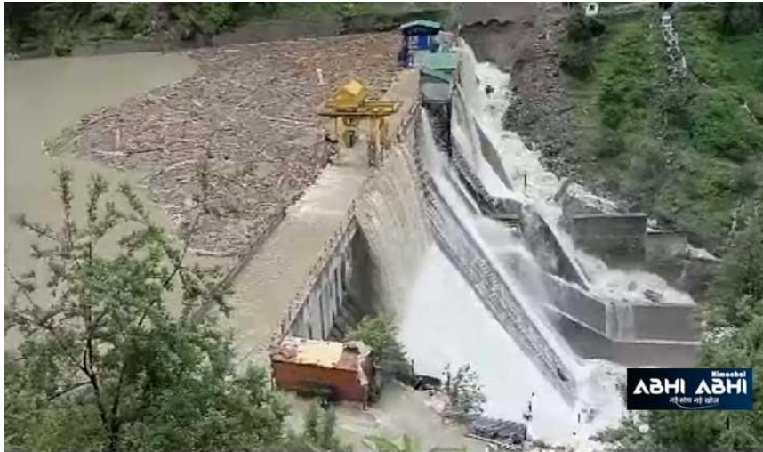
Sediment-laden flash flood caused a gate malfunction at the Malana Dam, leading to water overflow [18].
