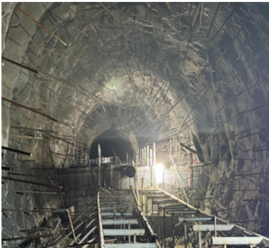
lining of DT3, DT3 Inlet and Exit Wing Wall Work
