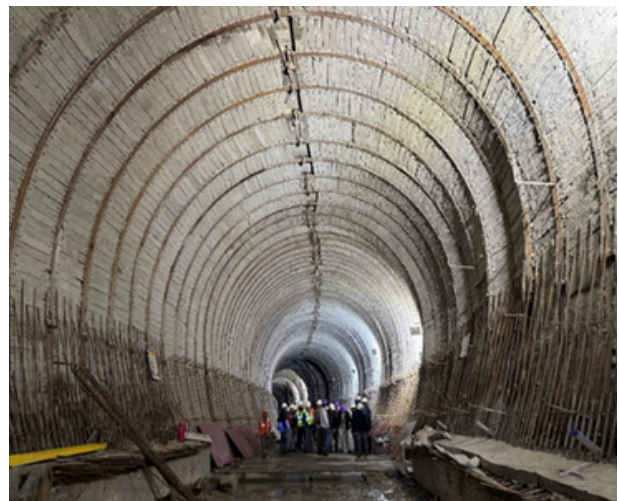
lining of DT3, DT3 Inlet and Exit Wing Wall Work
