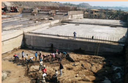
The construction of Garudeshwar Weir, 12 kilometres d/s of Narmada Dam will store one Million Acre Feet (MAF) water, 1/4th of the Narmada Dam's capacity. The water from the weir will be pumped back to generate power.
