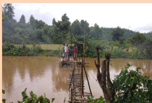
Diamond Core Drilling in River Bed at Proposed Dam Axis at Kharswati Irrigation Scheme Jharkhand
