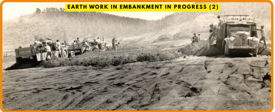
EARTH WORK IN EMBANKMENT IN PROGRESS
