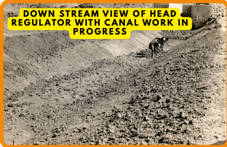
EXCAVATION OF CUT-OFF TRENCH IN PROGRESS
