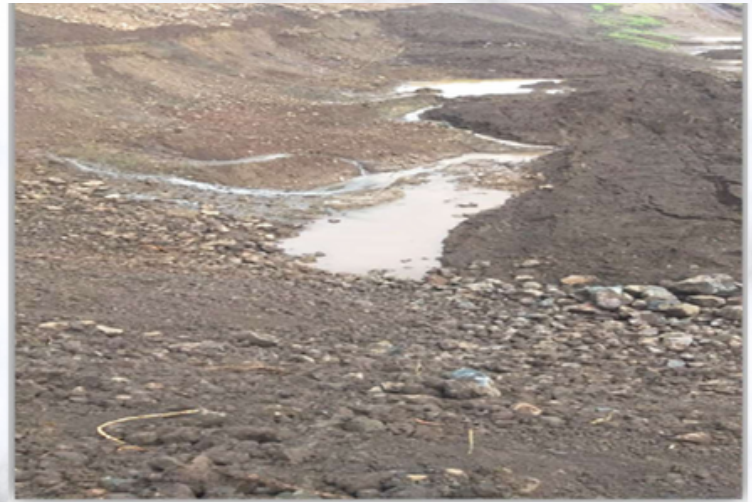
Fig.1- Downstream Slope Failure
