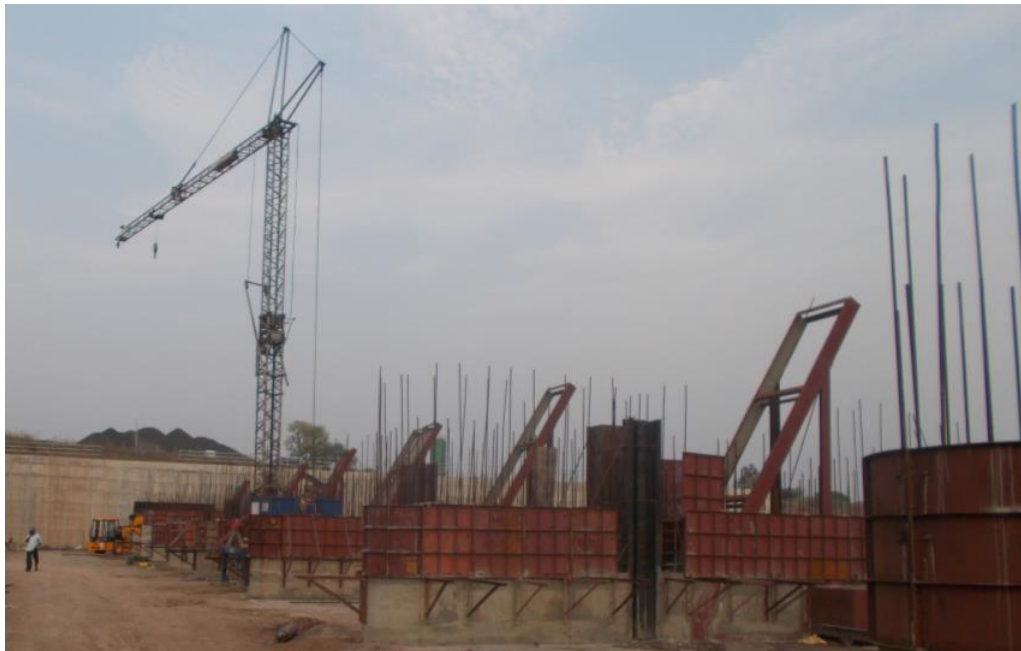
Erection of embedded parts of 10 m x 6 m size Automatic Gates on Marda Weir
