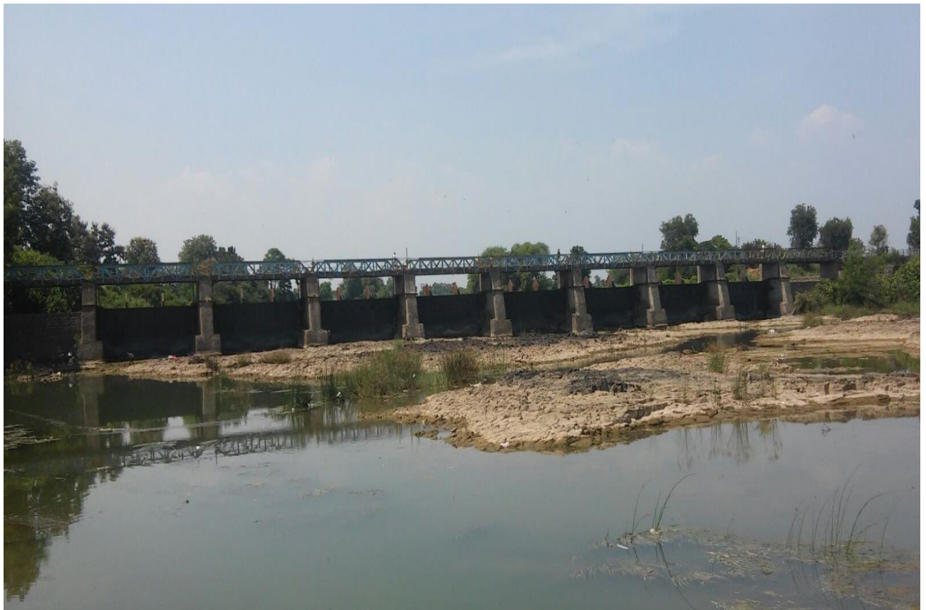
8 No. of 10 m x 4 m size Godbole Type Automatic Tilting Gates on Paunar Weir, Maharashtra.
