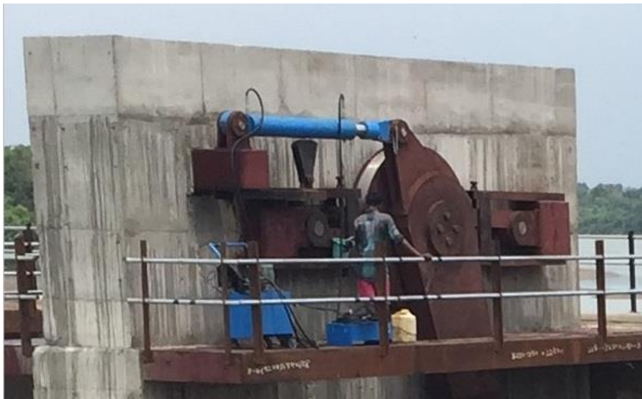
Emergency Hydraulic Hoisting Arrangement for Automatic Gates on Marda weir
