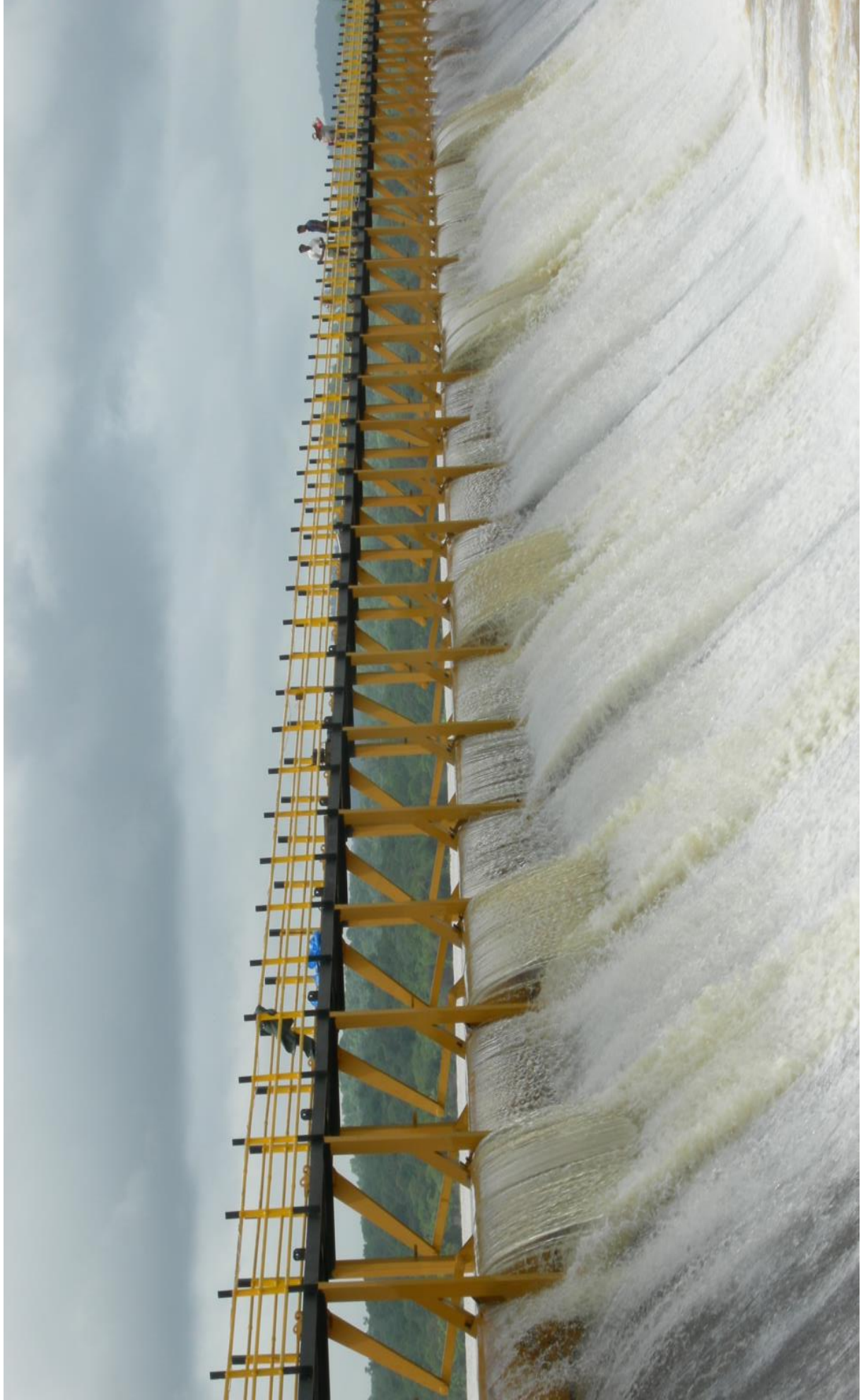
70 No. of 4 m x 1 m size Godbole Type Automatic Gates installed on Anjanpura Tank, Karnataka.
