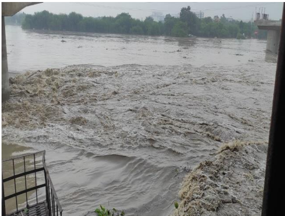
Photo 1: Delhi Railway Bridge during July 2023
