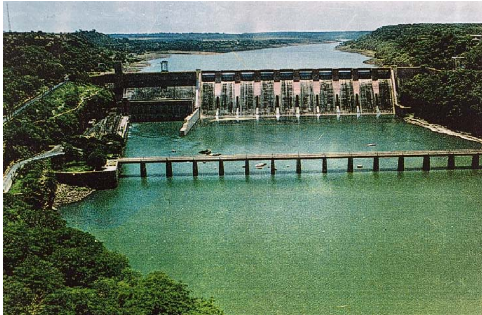
Photo 1: Spillway of Gandhisagar Dam and Power House as seen from downstream
