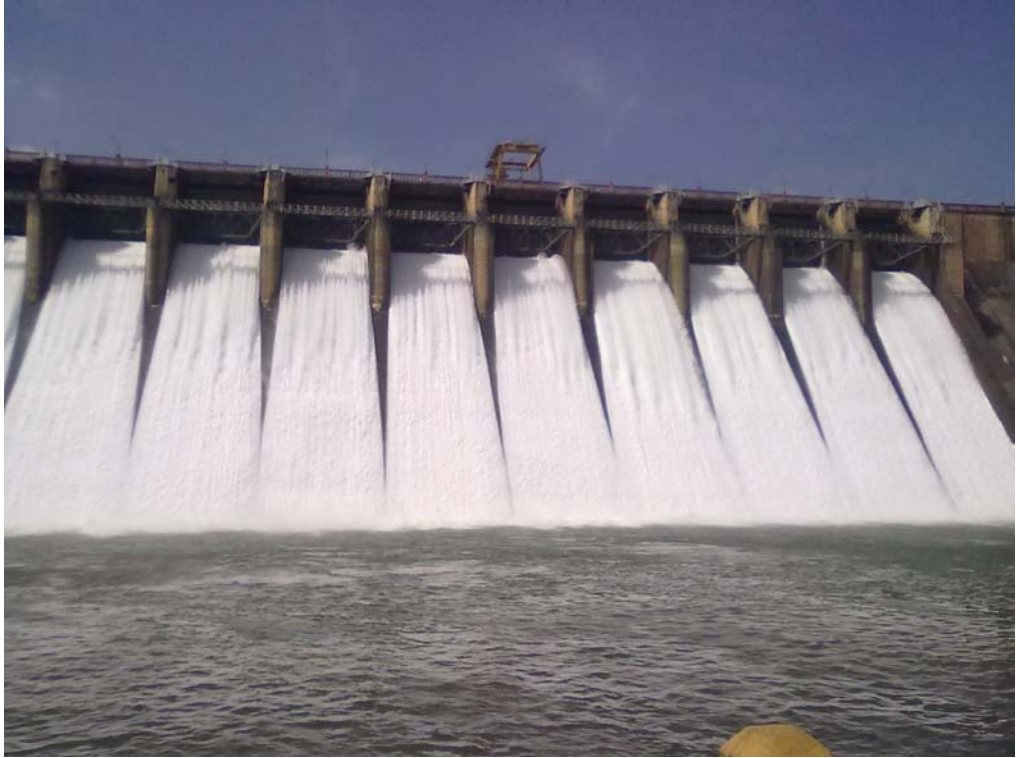
Photo 1 : Spillway of Ghatprabha Dam
