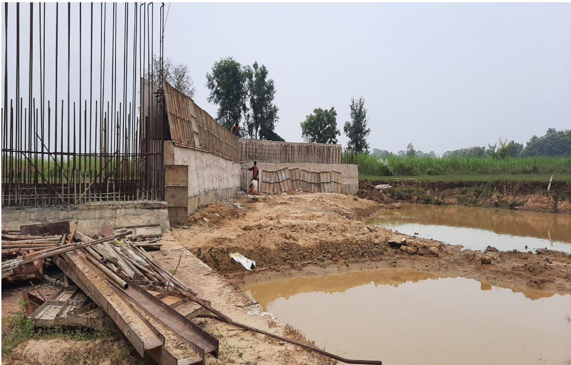
Syphon work under construction
