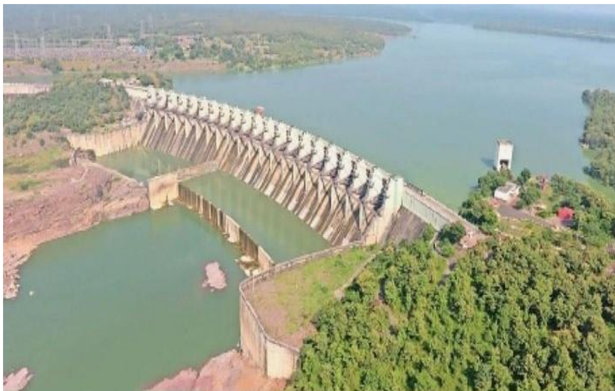
Photograph -6: Photograph of Indirasagar Dam, Khandwa.
