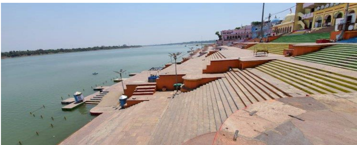
Photograph -2: Photograph of Sethani Ghat, Narmadapuram
