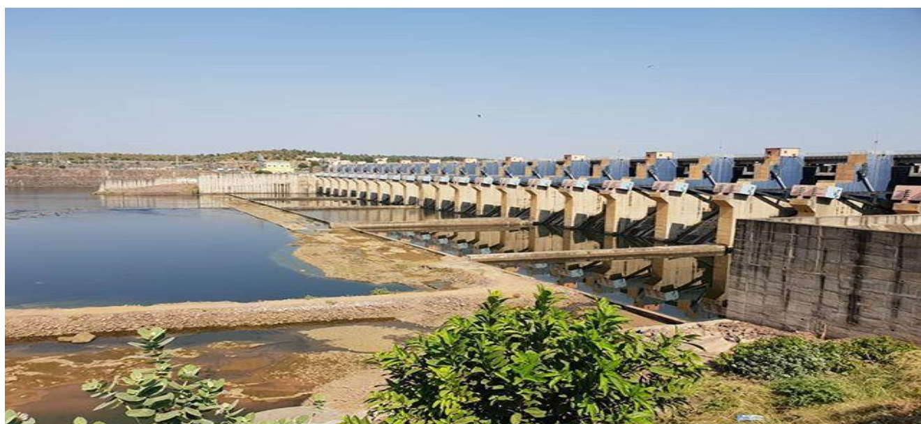
Photograph -7: Photograph of Omkareshwar Dam, Khandwa
