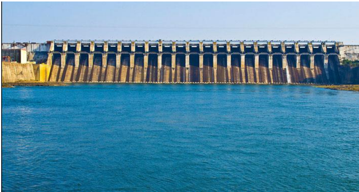
Photograph -3: Photograph of Bargi Dam, Jabalpur.
