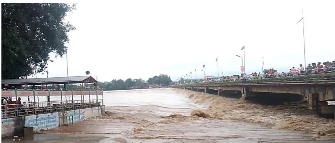
Photograph-1: Photograph of Rapti Ghat, Mandla during Flood.
