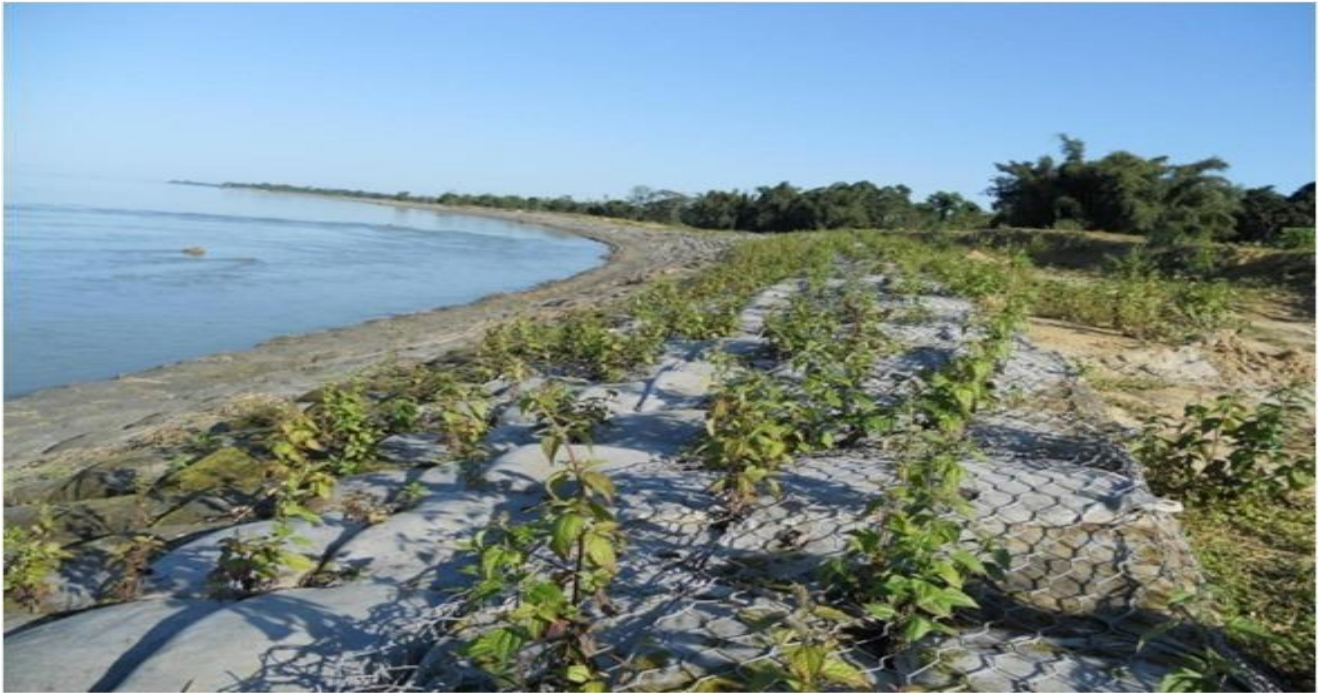
Bank revetment using geo bags at Rohmaria, Assam
