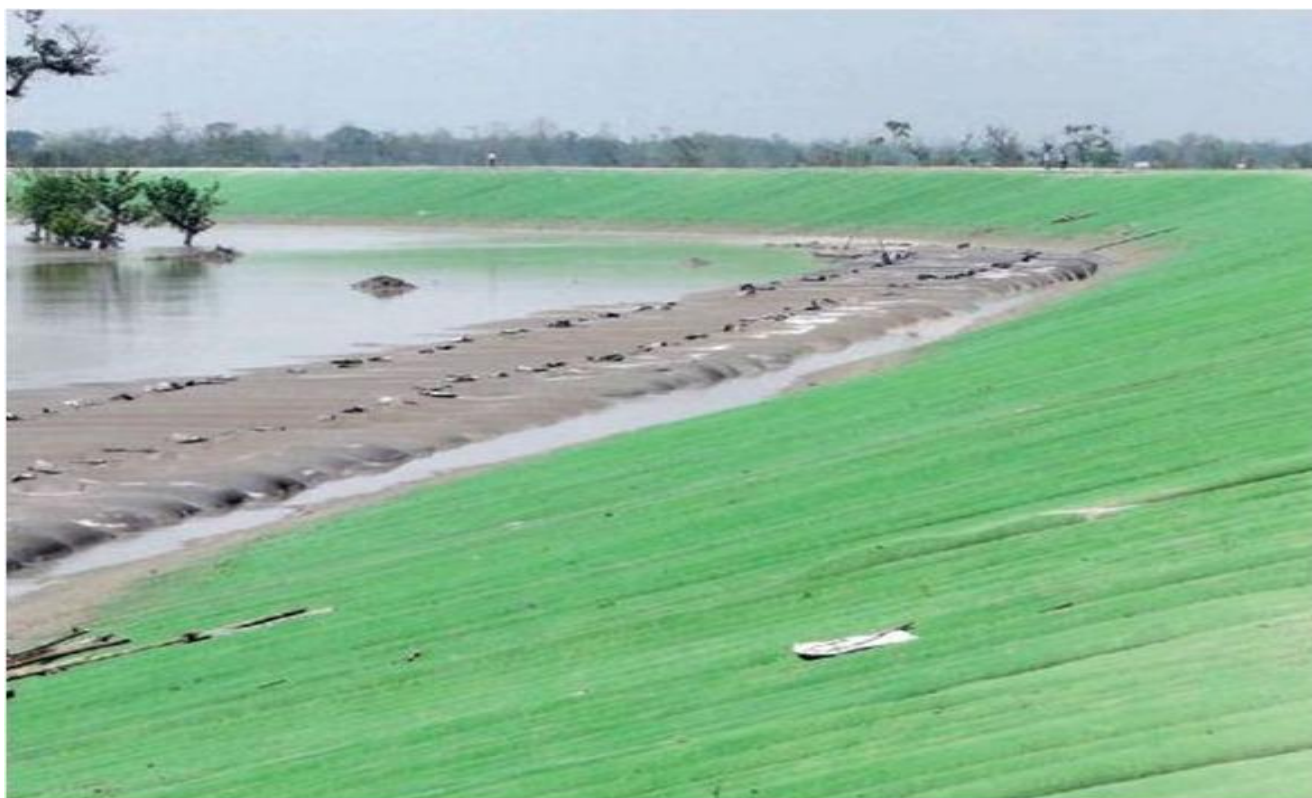
Embankment using Geo-tubes and Geo-mattress at Matmara, Assam
