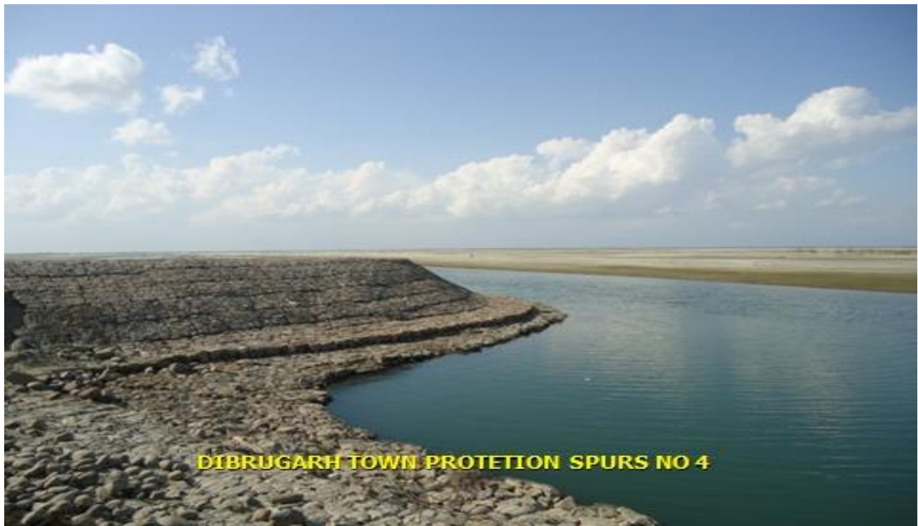
Protection with boulder Spurs at Dibrugarh, Assam
