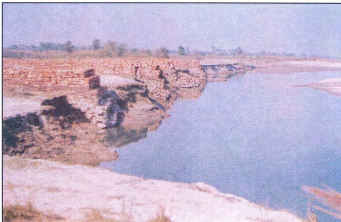
PHOTO 4: DAMAGED SPURS WITH STONE PITCHING
