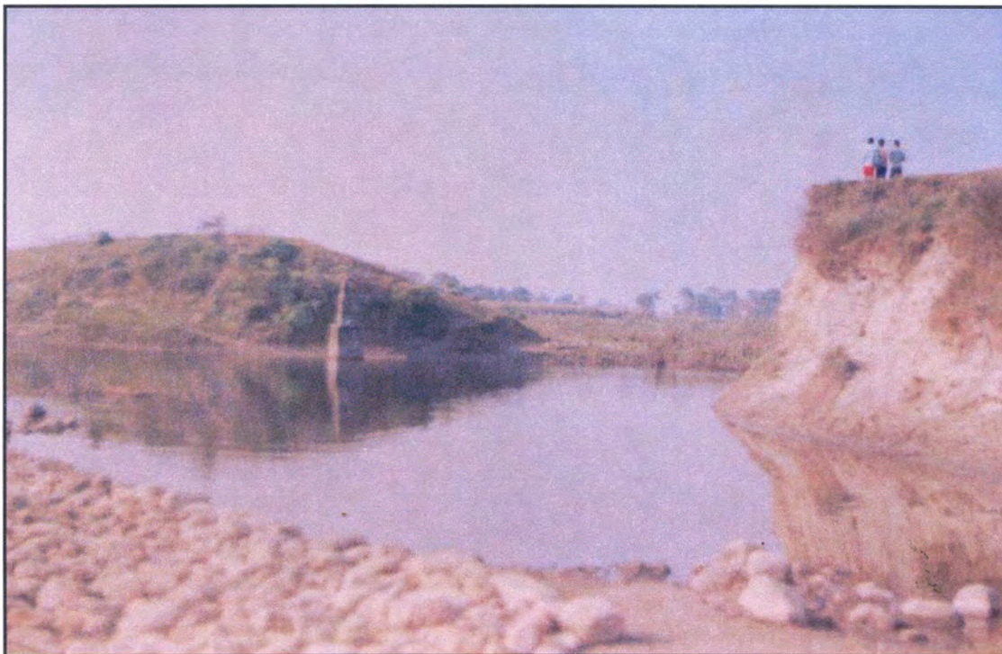
PHOTO 2: BREACH IN EMBANKMENT OF RIVER GANDAK
