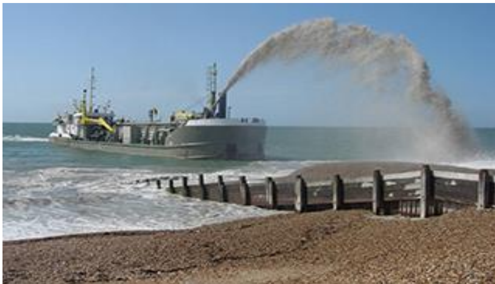
Beach Nourishment – Softer solution for protection
