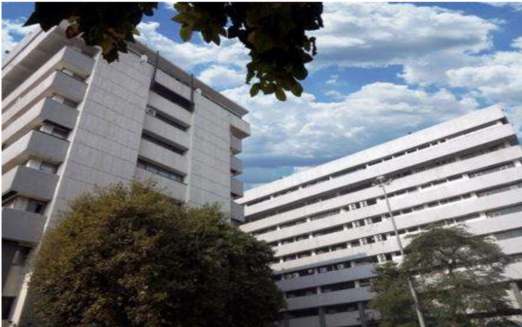
CENTRAL WATER COMMISSION (HQ), SEWA BHAWAN, R K PURAM, NEW DELHI
