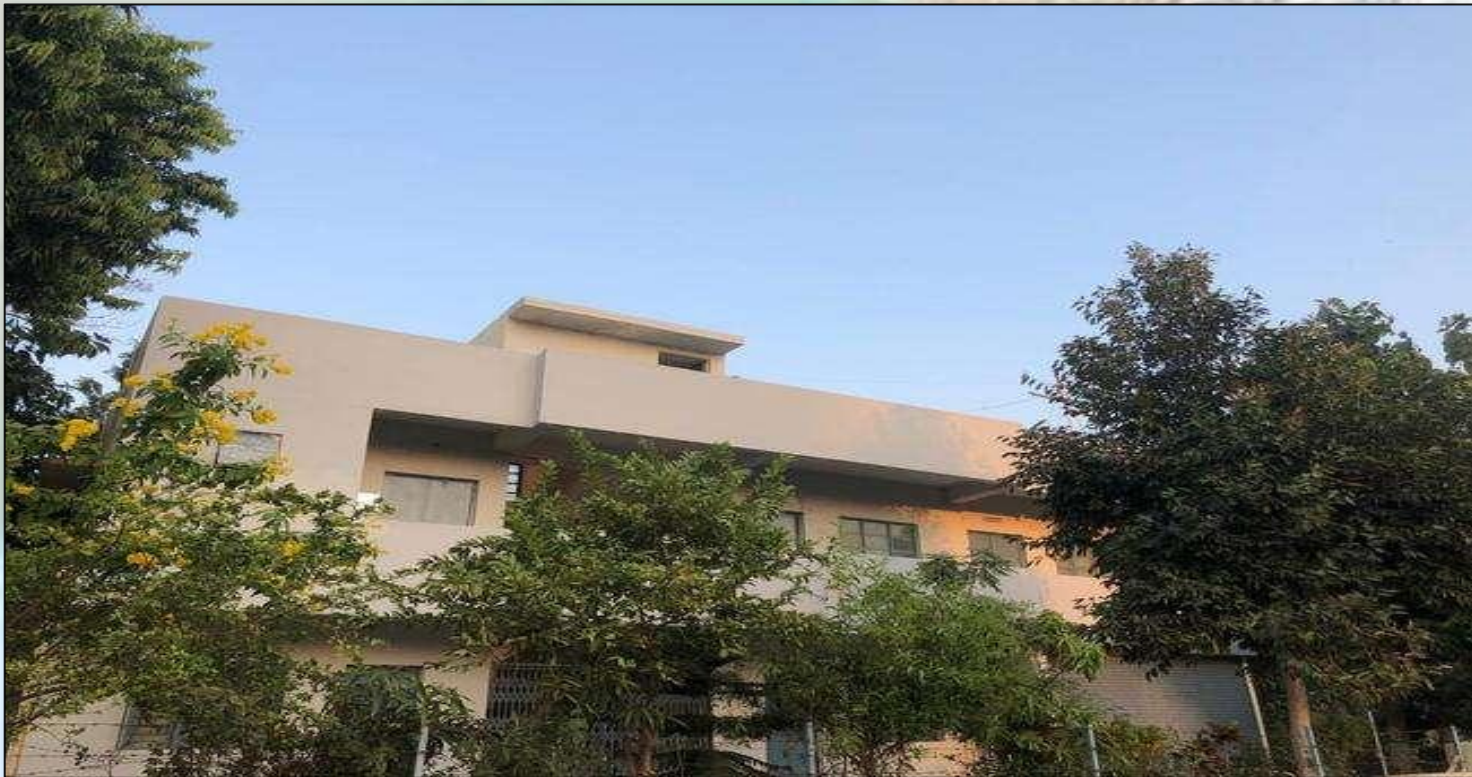
NORTH WESTERN RIVER SUB DIVISION. HIMMATNAGAR
