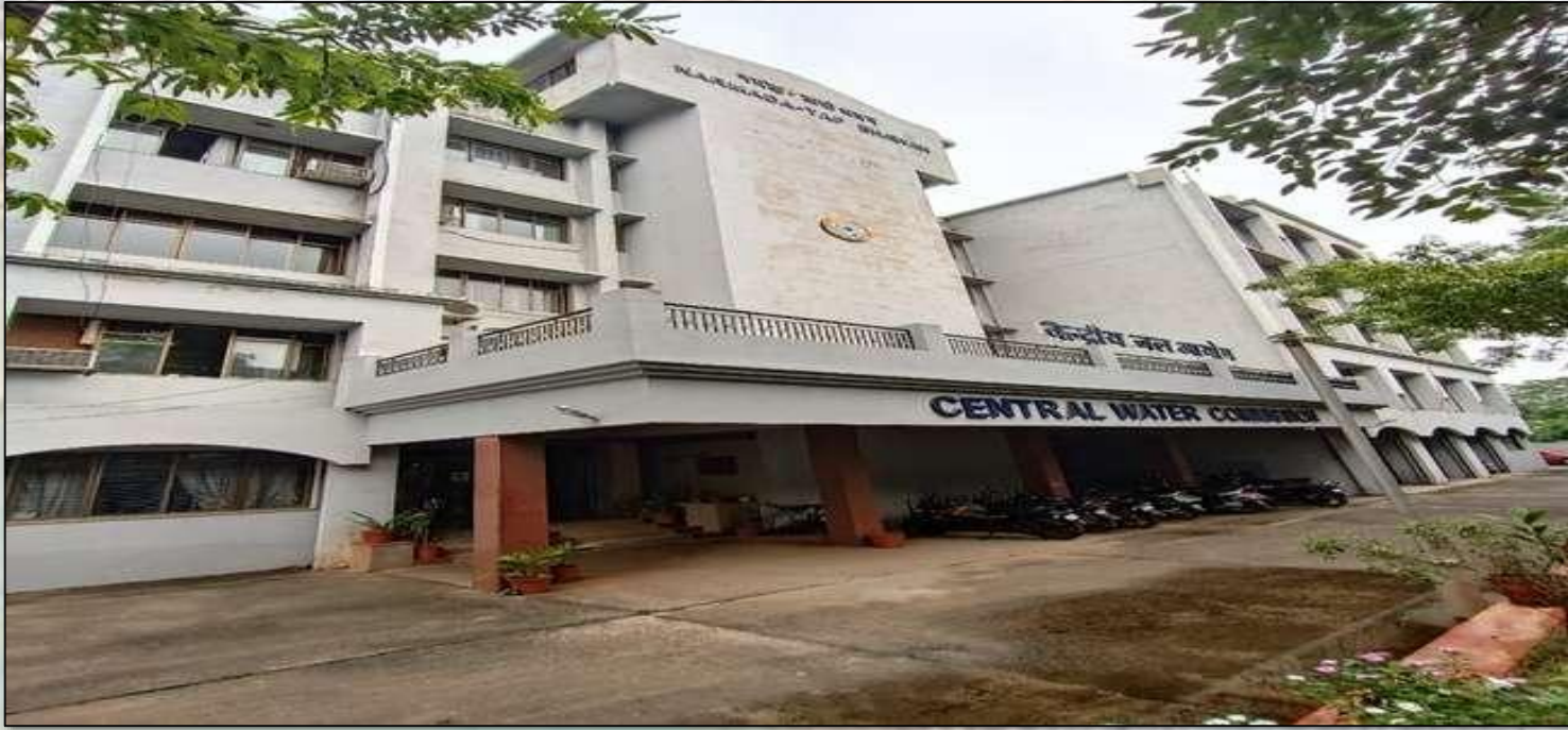
NARMADA TAPI BHAWAN BUILDING
