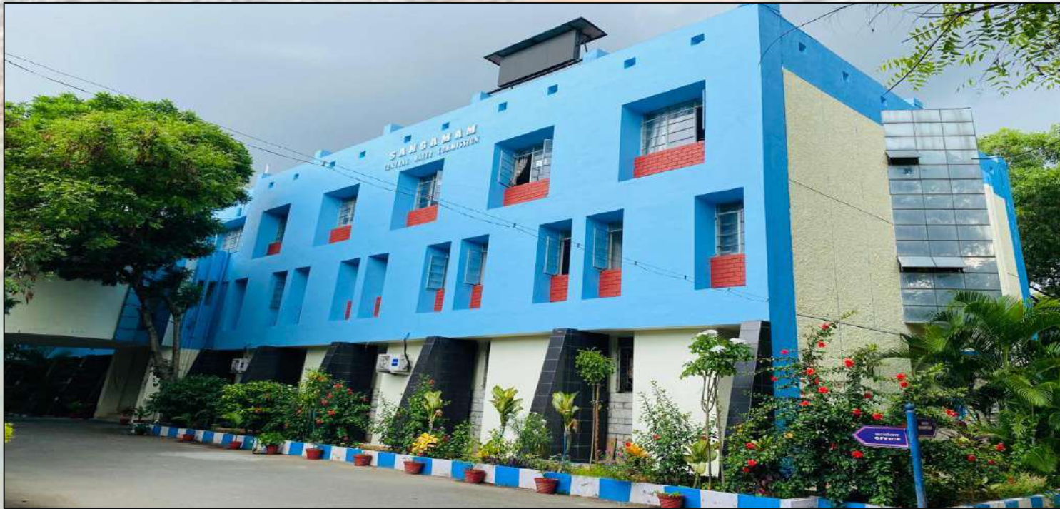
“SANGAMAM” OFFICE BUILDING OF CWC AT COIMBATORE
