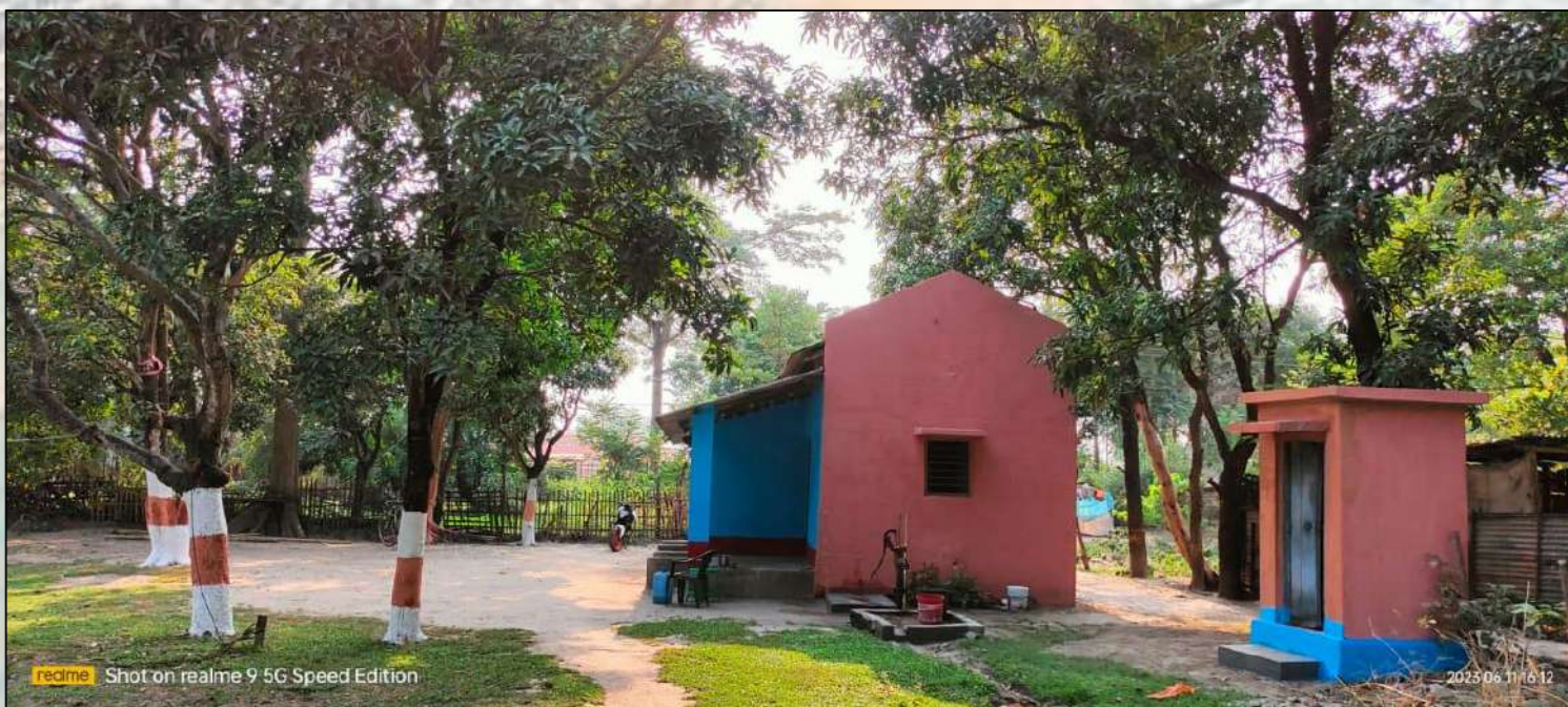
BIRPUR GAUGE SITE ON KOSI RIVER, LOWER GANGA DIVISION-1
