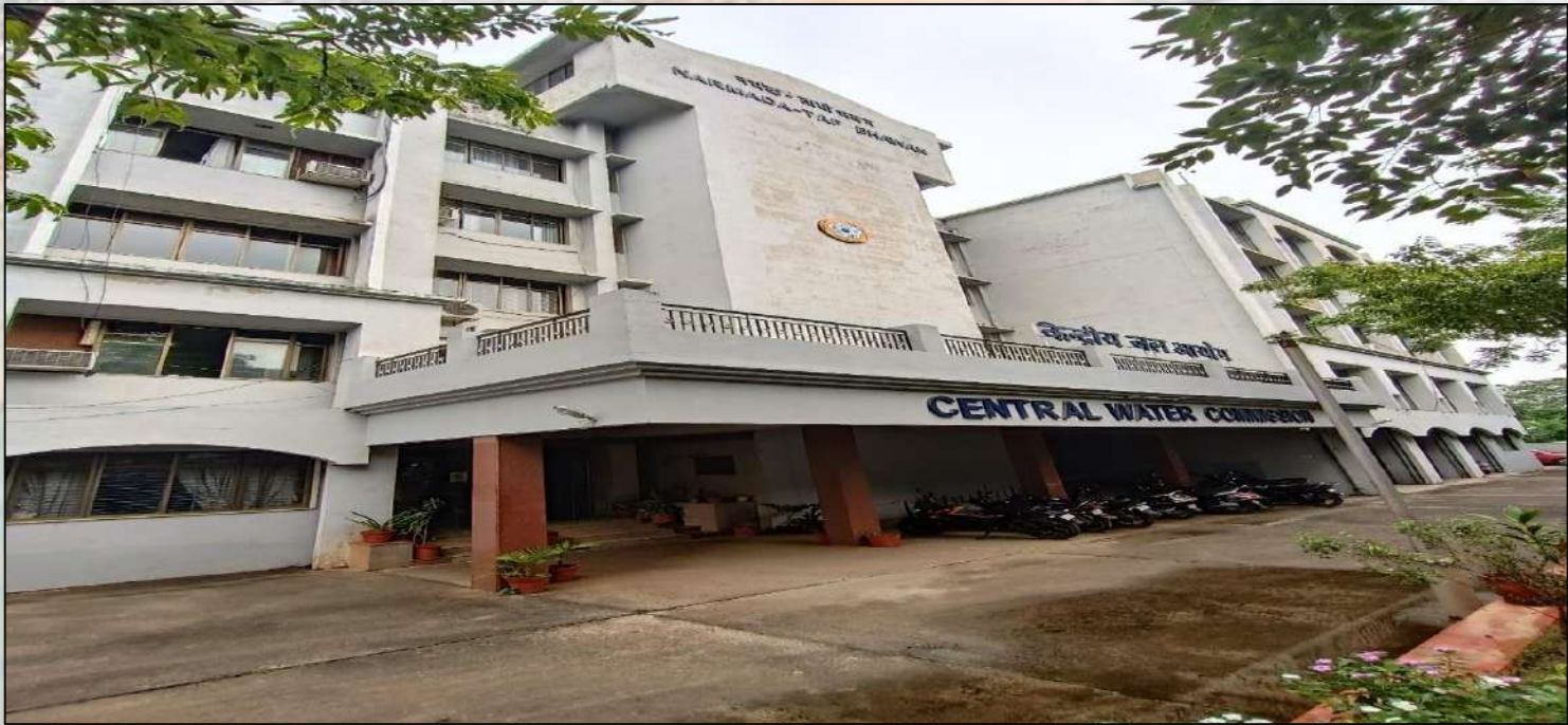
NARMADA TAPI BHAWAN BUILDING
