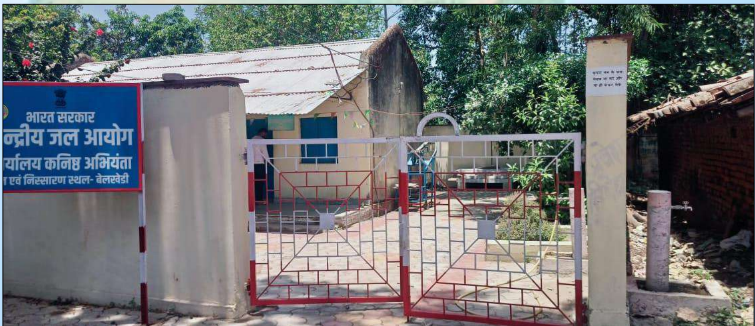
SITE OFFICE- BELKHERI ON SHER RIVER UNDER, NARMADAPURAM
