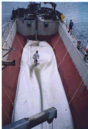
SPLIT HULL HOPPER DREDGE FILLING SANDBAG
