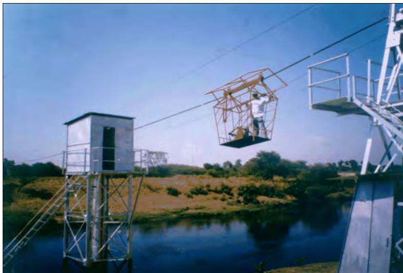
Figure 6.30: Cableway with manned trolley
