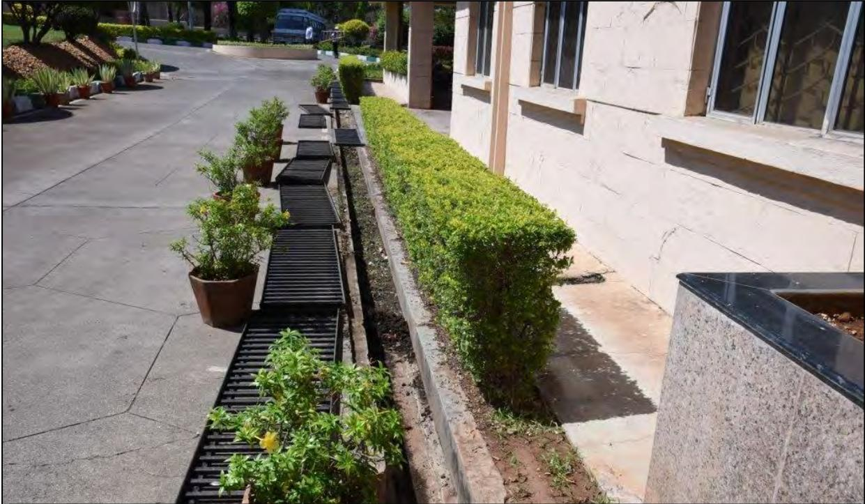
**Figure 8A: Silt, dirt and dried leaves had clogged the NWA Campus Storm Water Drains thereby reducing their capacity resulting in water logging during torrential rain.**
