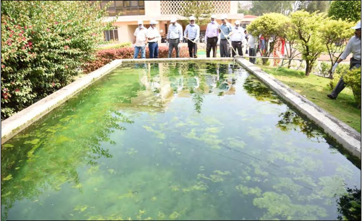
**Figure 5A. Tank of NWA for storing pumped out Ground Water (GW), full of algal growth.**
