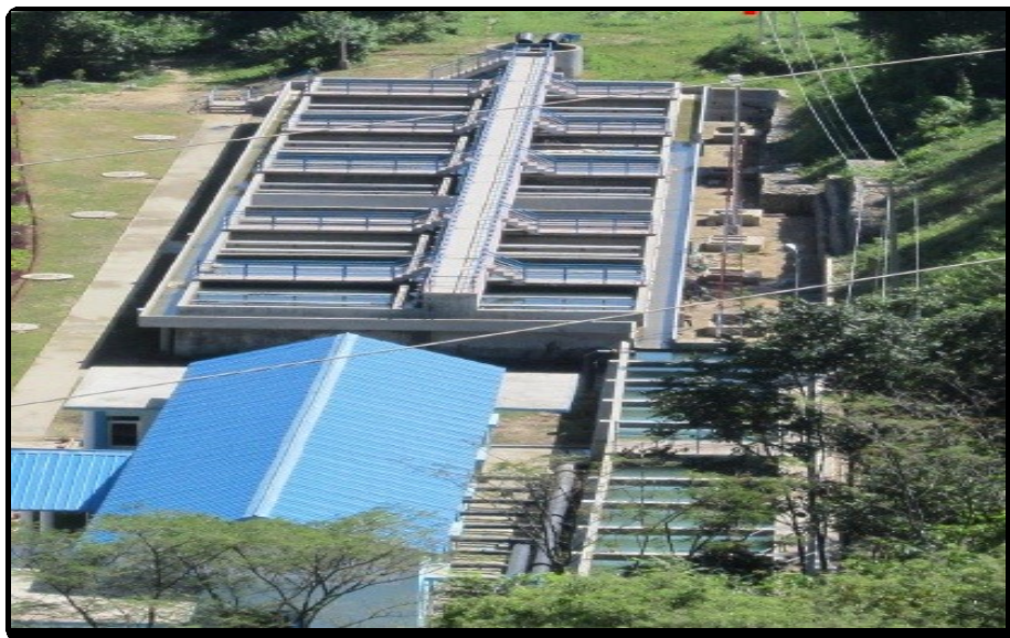
Figure 6.16 Aerial View of Tube settler type desilting arrangement provided in Balh Valley Medium Irrigation Project, HP
