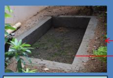
Rainwater Harvesting structures of infiltration capacity around 7 cum
