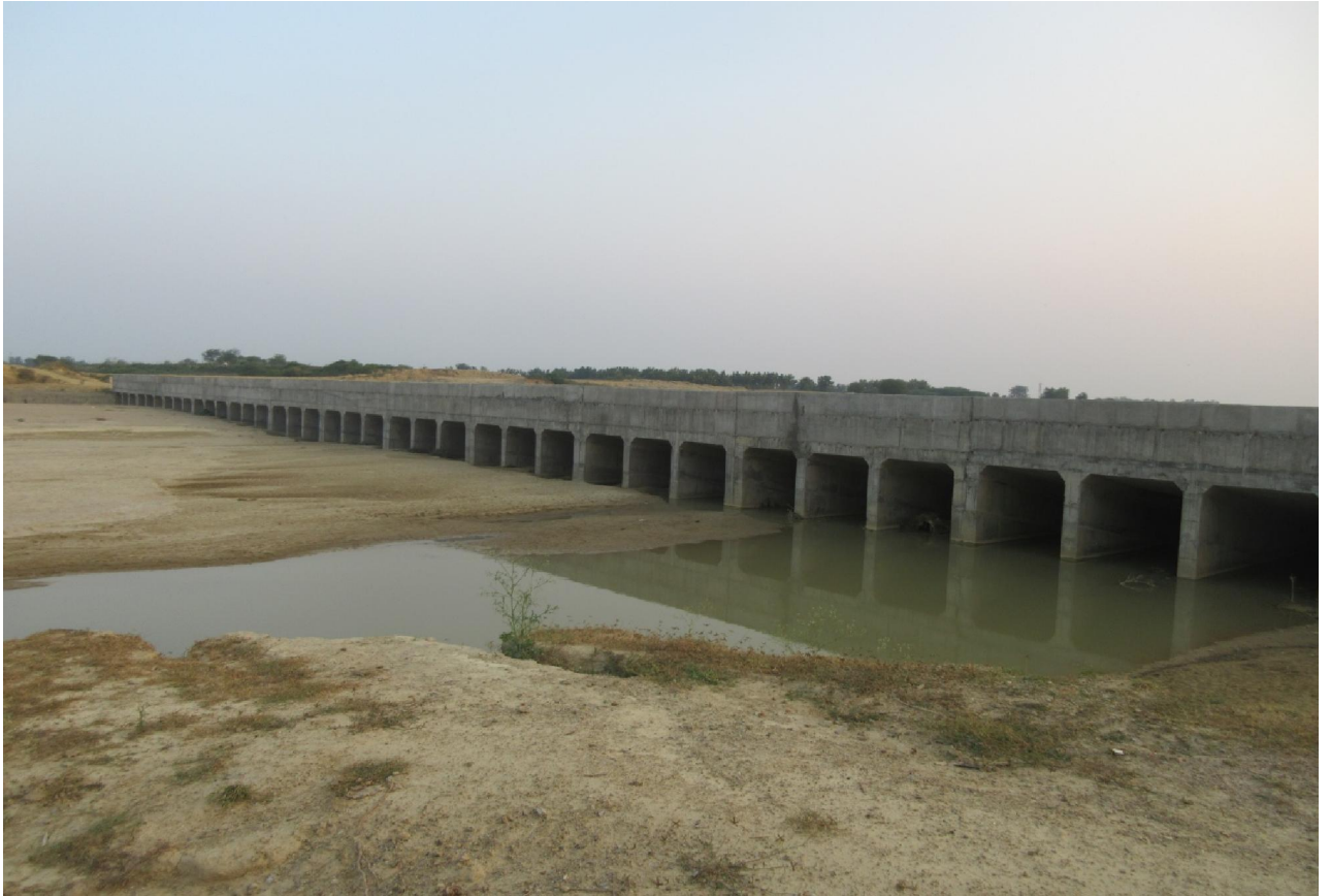
Drainage siphon at Km. 87.200 of Rapti Main Canal
