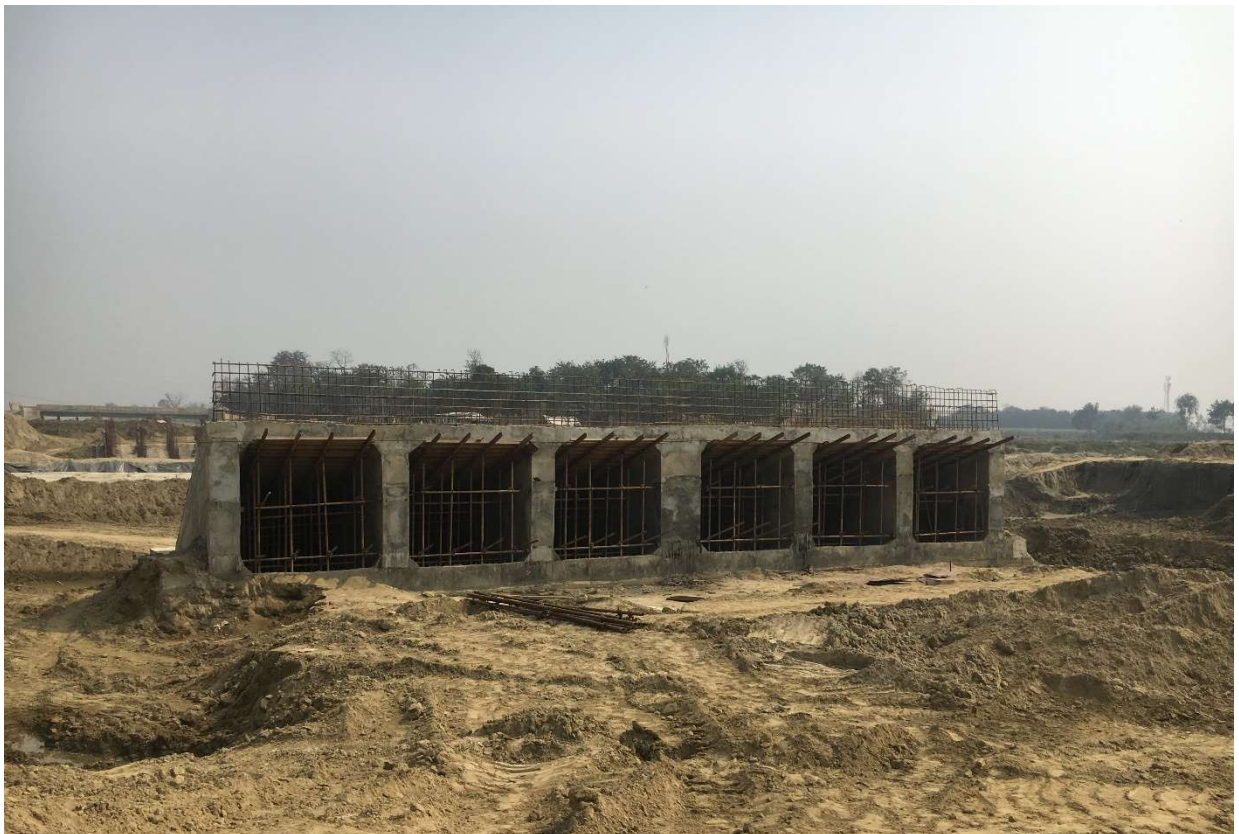
Drainage syphon at km 112.130
