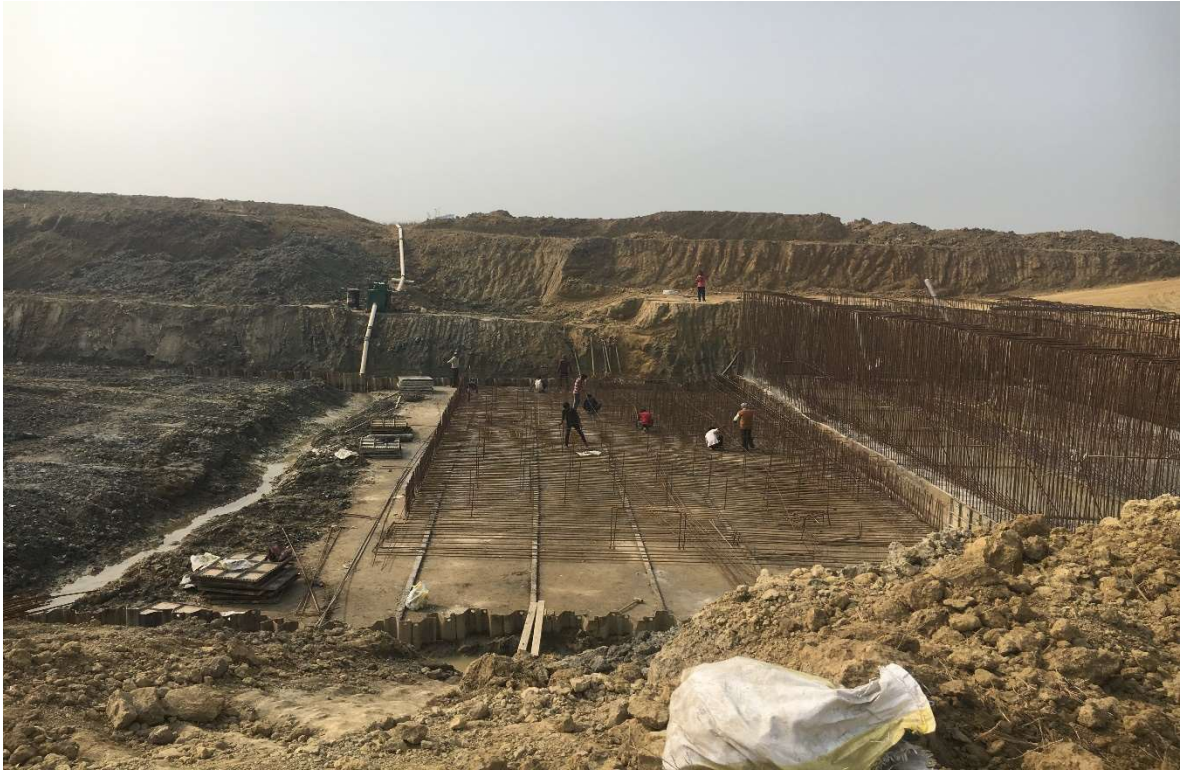
Drainage Syphon at km 32.829
