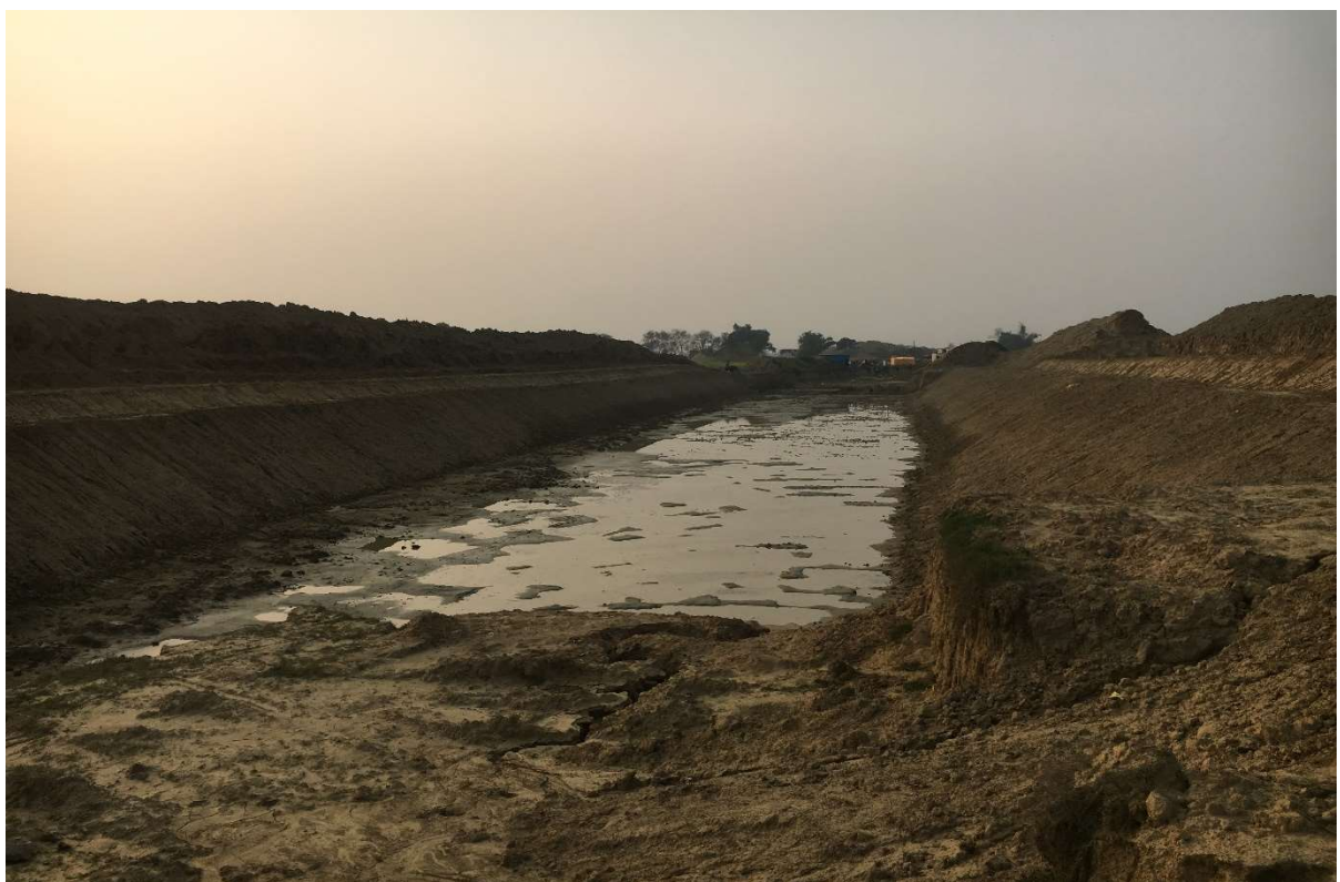
Earthwork of the off taking Brijamanganj distributary
