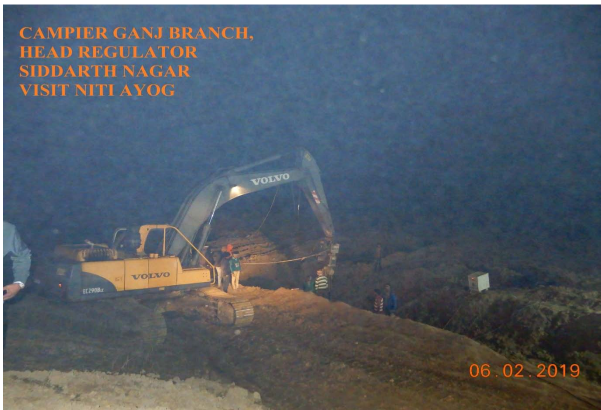
Trench digging work under progress for cut-off wall fo Headworks of Campiergang branch
