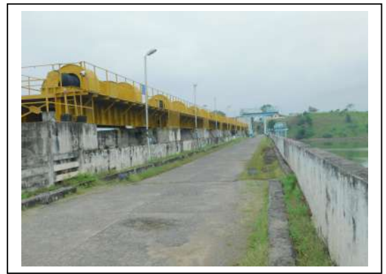
Top bund level
