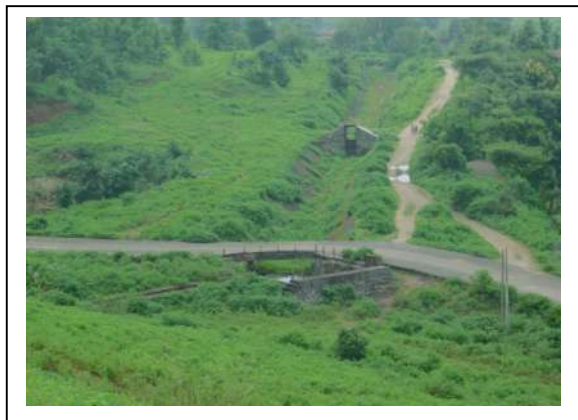
Left bank canal
