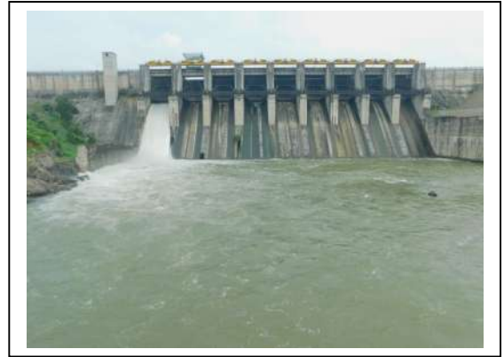
Downstream side of dam
