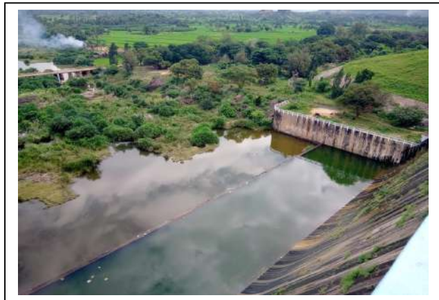
Energy dissipation arrangement of dam
