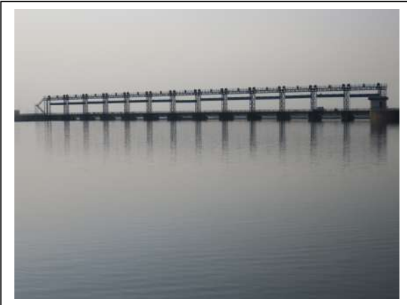
Overflow section with gates
