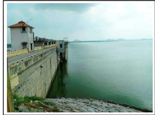
Dam upstream side
