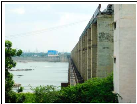
Dam downstream side
