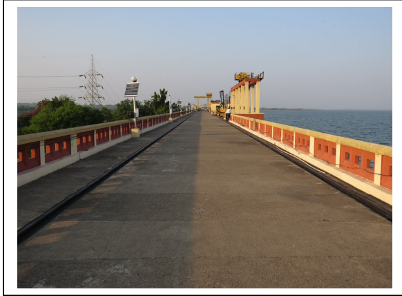
Top bund level
