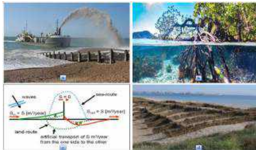
Fig. 3 (a) Artificial nourishment of beaches (b) Coastal vegetation such as mangrove and Palm plantation (c) Sand bypassing at tidal inlets (d) Dune reconstruction/rehabilitation
