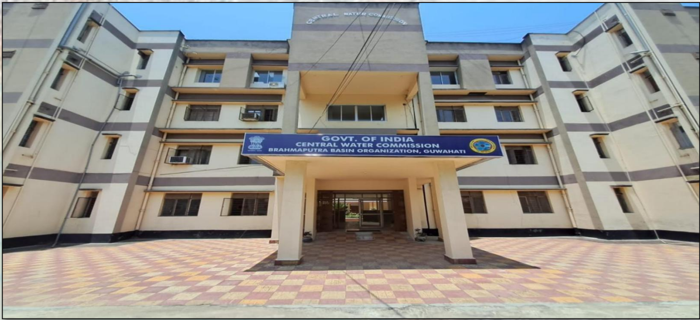
BBO OFFICE COMPLEX, ADABARI, GUWAHATI
