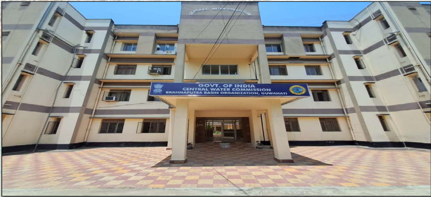
BBO OFFICE COMPLEX, ADABARI, GUWAHATI
